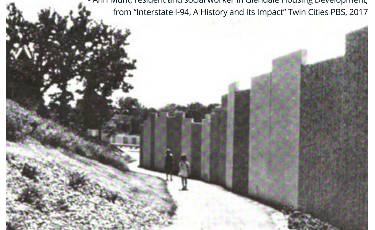
Figure 4. Concrete Noise Wall on I-94 in Prospect Park, Minneapolis Source: Minnesota Highways October 1974 - Haihi Trust.jpg
