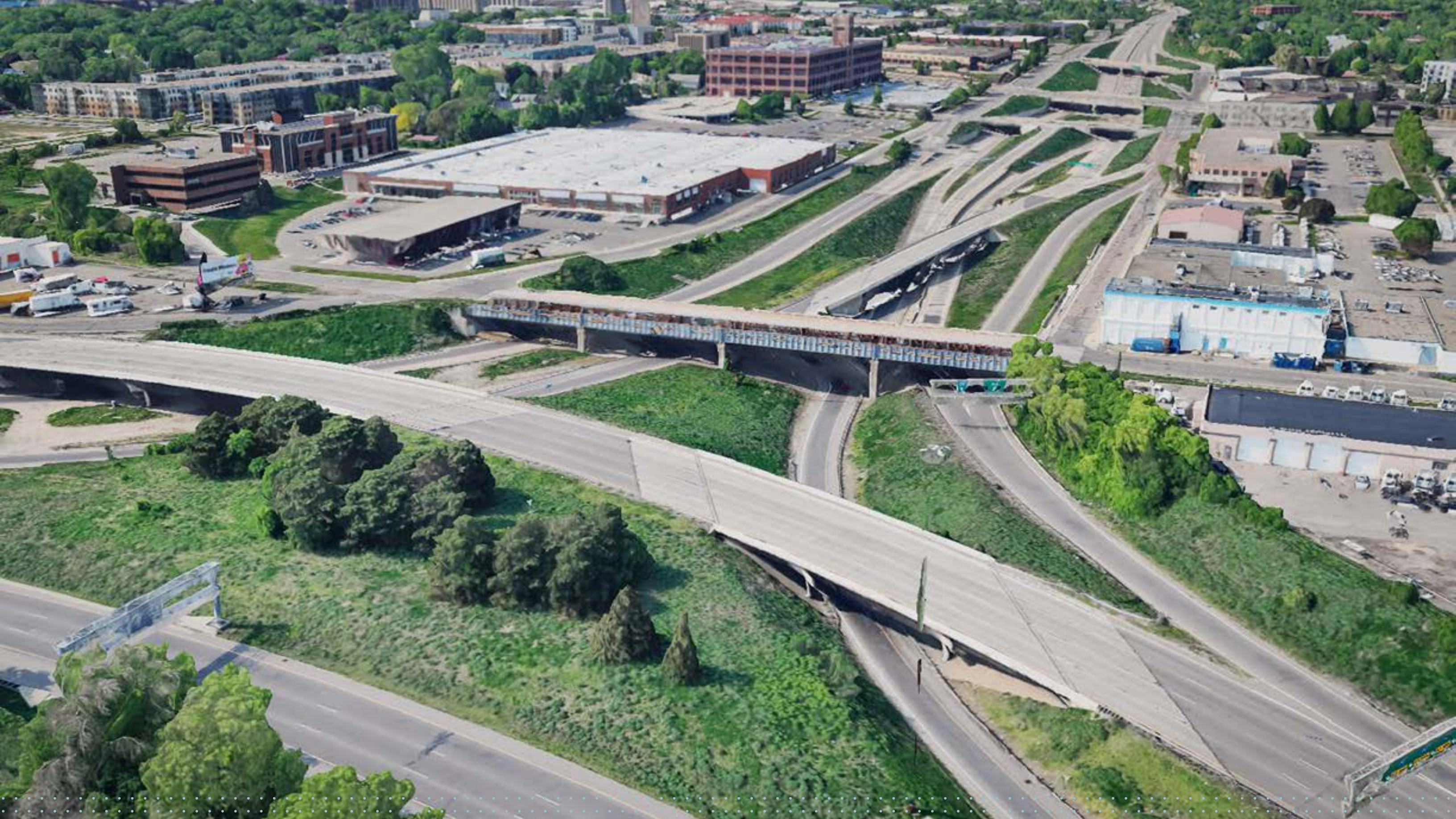
Highway 280 interchange with I-94, with an arrow of grade separated on- and off-ramps.
