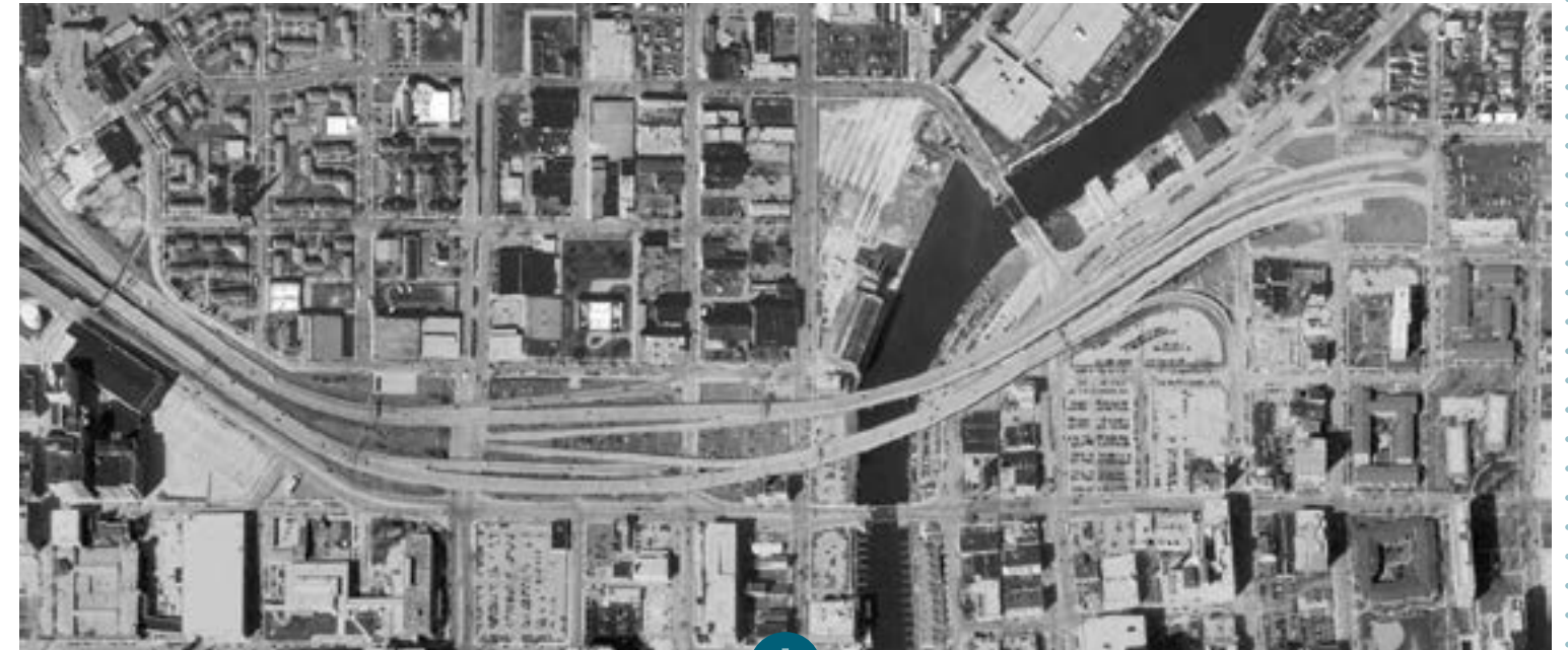
Figure 36. Progression of the Park East Freeway Removal. Source: Google Earth
