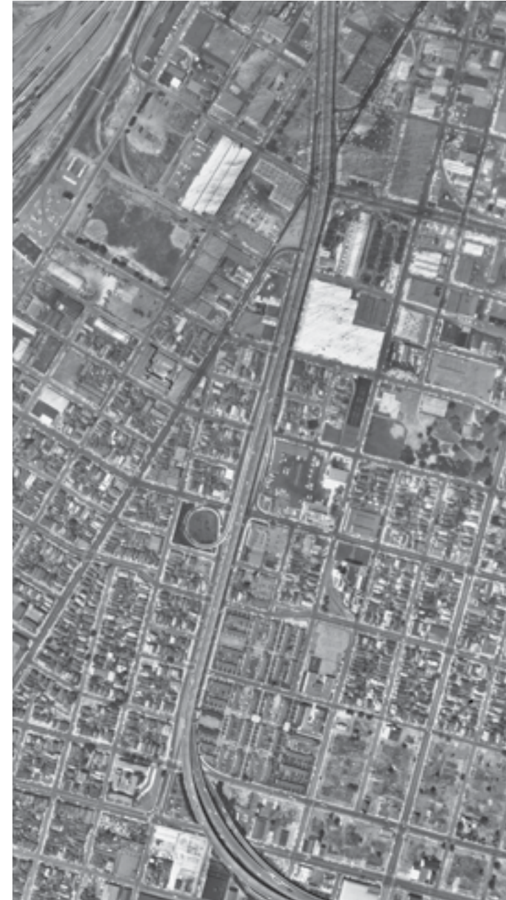
Figure 37. Aerial of the Cypress Street Viaduct before it fell down. Source: USSB Archive
