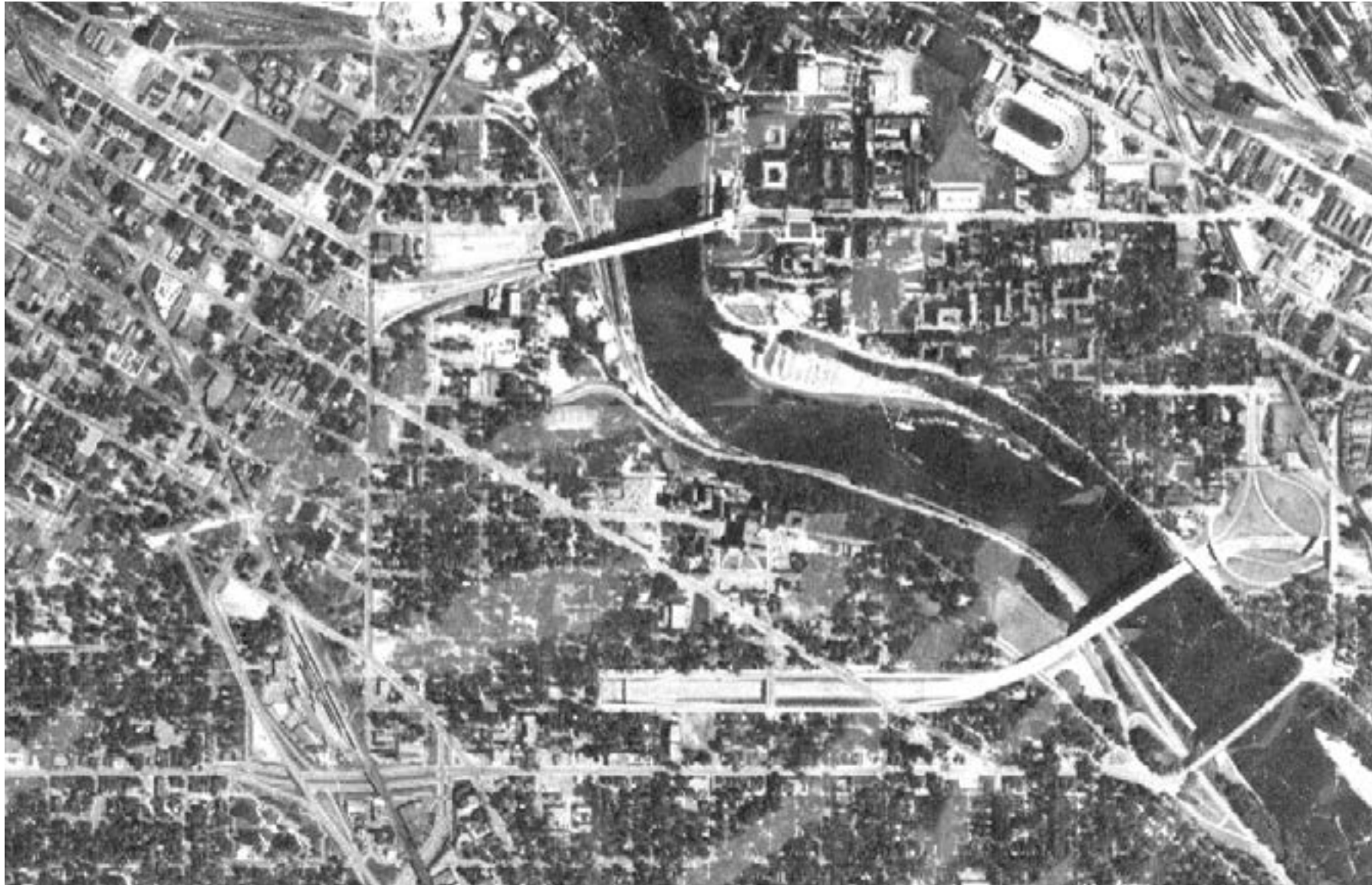
Figure 3. 1966 aerial highway under construction through Cedar-Riverside. Source: Hennepin County Libraries.
